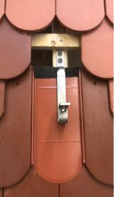
If the plain tile collides with the roof hook, push the tile up a
